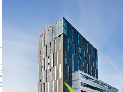
Eurocity Center West, Mannheim
