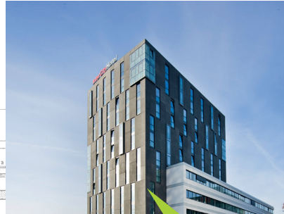
Eurocity Center West, Mannheim
