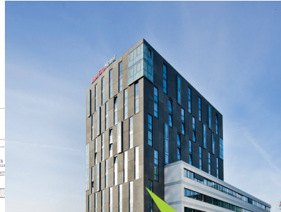
Eurocity Center West, Mannheim
