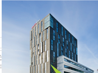
Eurocity Center West, Mannheim
